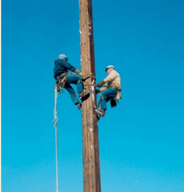
E-LAM ® is the only engineered pole which can be climbed with hooks and drilled with standard tools.
