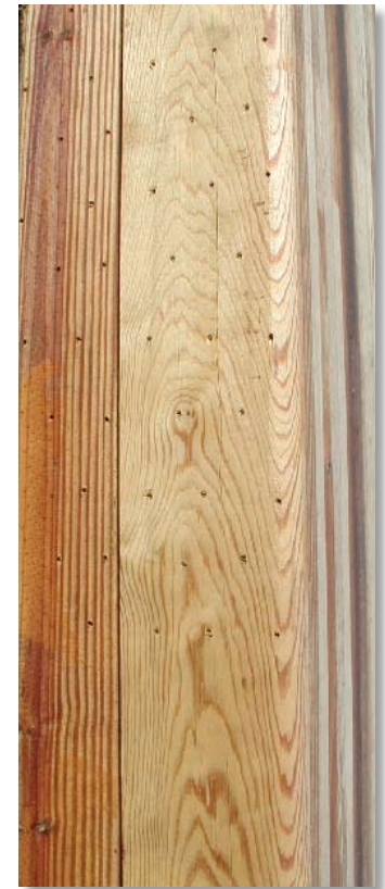
Groundline deep boring.
