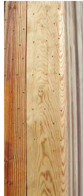
Groundline deep boring.
