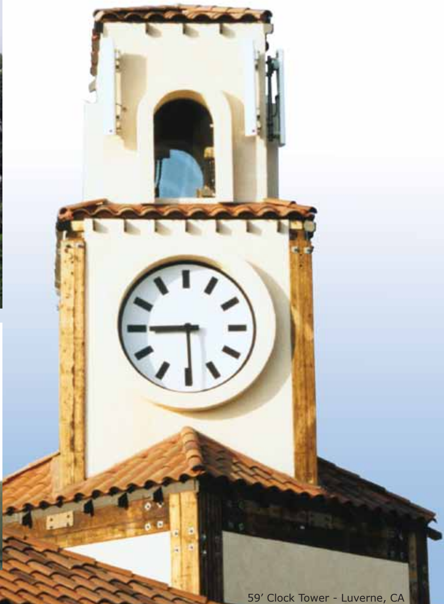
59' Clock Tower - Luverne, CA
