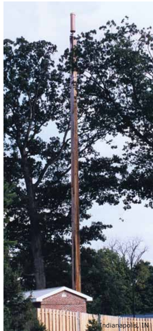
■ MONO POLE TOWER
