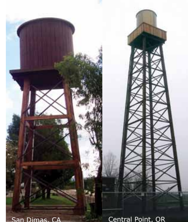
■ WATER TOWER STRUCTURES
