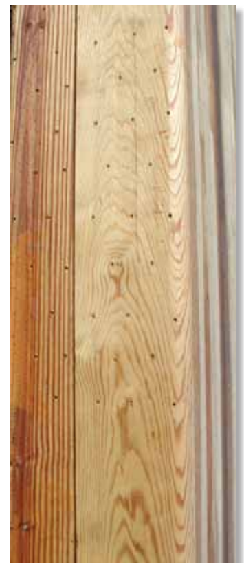
Groundline deep boring.
