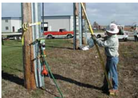
Raise Hammer Assembly approximately 3 feet.
