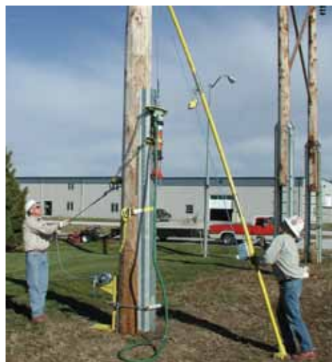
Raise Air Hammer to top of steel using Winch Pole.
