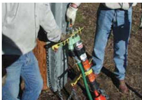
Attach winch line to Hammer Assembly.
