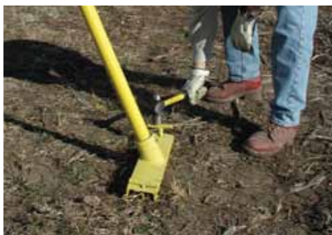
Secure Winch Pole Assembly base by driving two “T” Pins into the ground.
