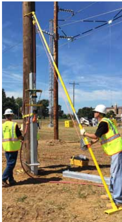
1. Lower steel unit is driven next to pole.
