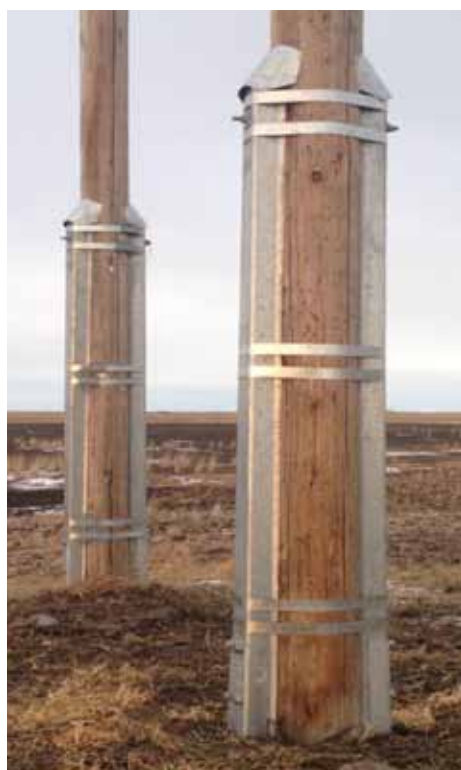
6. Units are banded and caps are installed.
