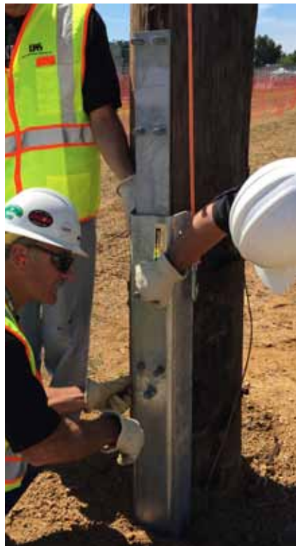
2. Back splice plate is attached to the lower steel unit.
