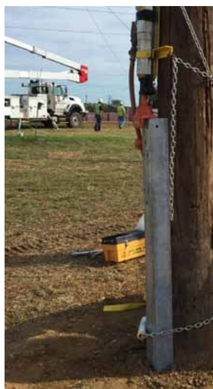
5. Steel SRS units are driven to desired depth.
