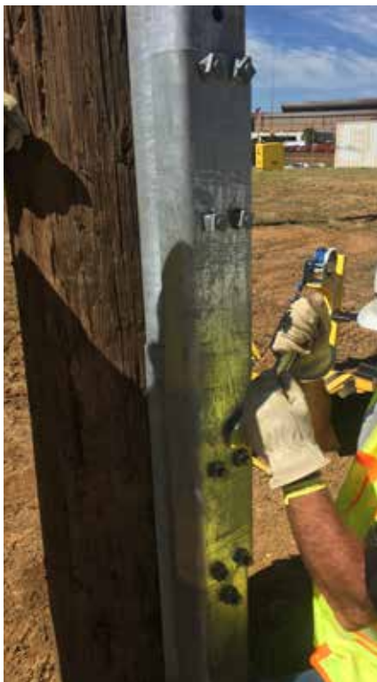
4. Splice channel is attached and secured with nuts and locknuts.
