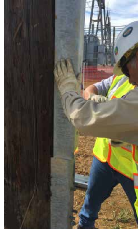
3. Upper steel unit is positioned on top of lower unit.
