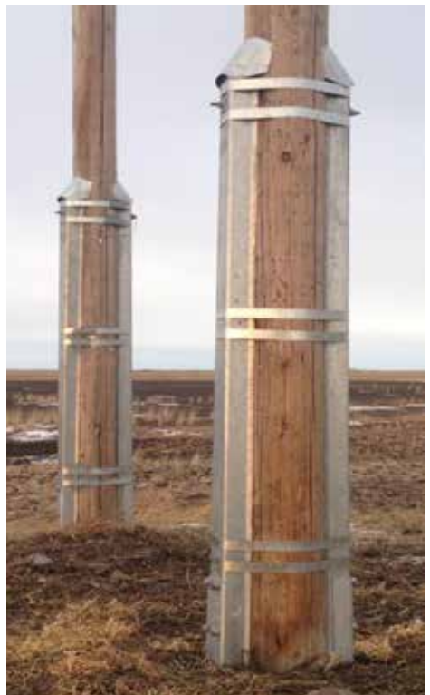
6. Units are banded and caps are installed.
