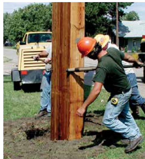
Adjust and align structure using a cant hook or similar tool.
