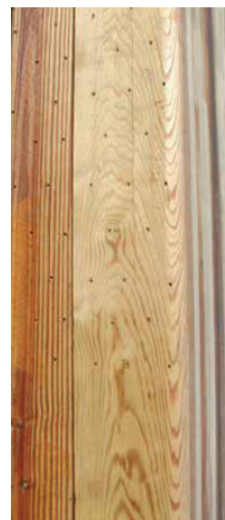
Groundline deep boring.
