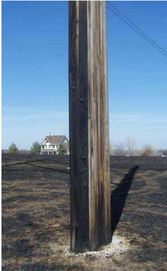
E-LAM® laminated wood structure after a grass fire shows minimal char and less than 1% reduction in strength.
