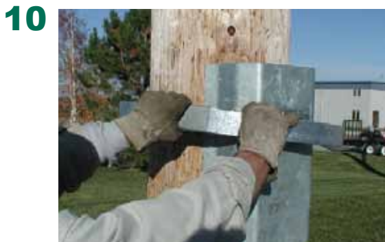
10 Wrap Banding around pole / steel and slide the uncurled end through Seal as shown.
