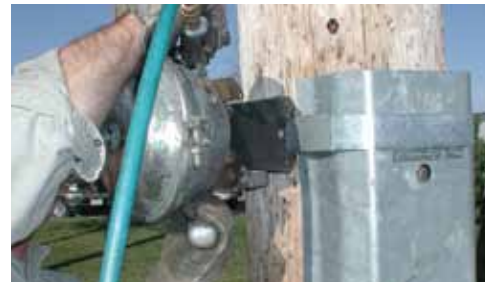
13 Apply 4 crimps to the Seal using either an Air or Manual Crimper.†
