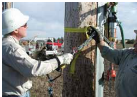
Attach Bridal Roller to the hammer chain bridals free-floating sling links.
