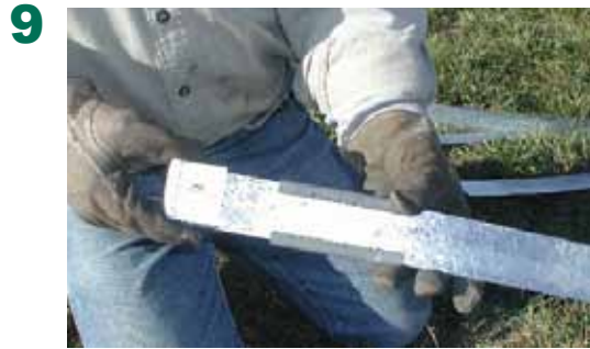
9 Make sure the Seal is oriented as shown, with the open side toward the curl.
