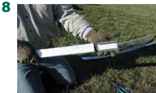
8 Slide a Seal onto a piece of Banding.
