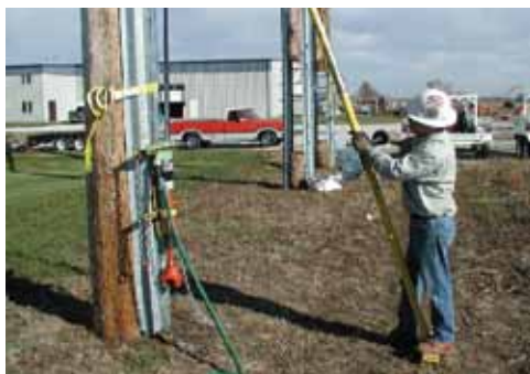
Raise Hammer Assembly approximately 3 feet.
