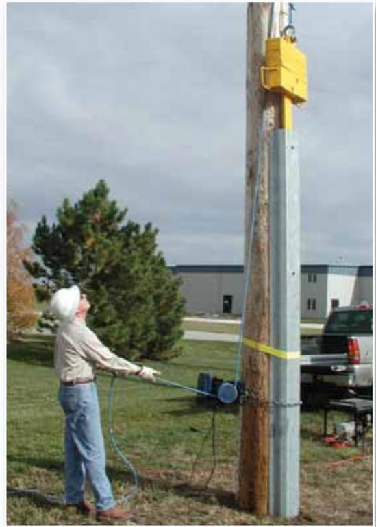
Pneumatic and drop weight driving systems are available as well as a full line of specialized tools. Payback on the initial tool cost is realized after only a few installations.
