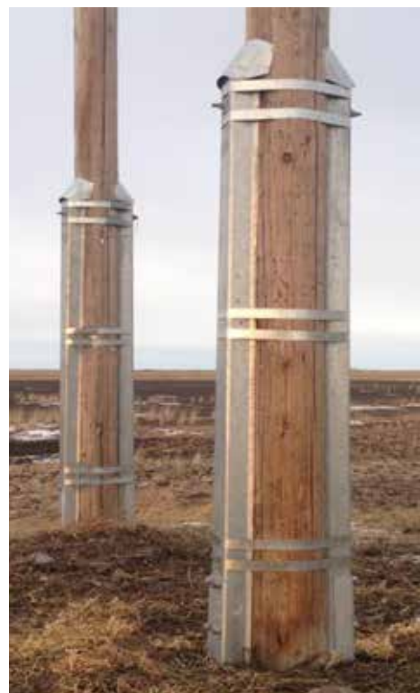
5. Units are banded and caps are installed.
