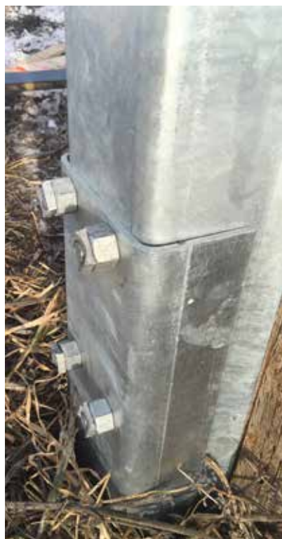
4. Assembled units are driven to desired depth.
