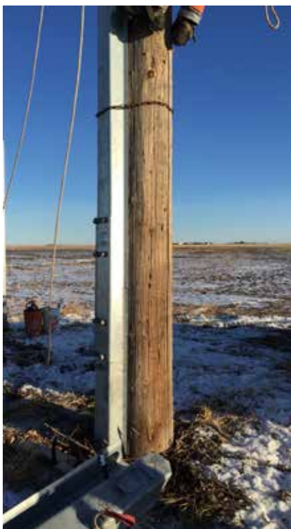
4. Assembled units are driven to desired depth.
