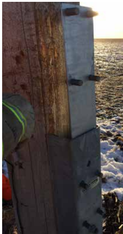
2. Back splice plate is attached to the lower steel unit.
