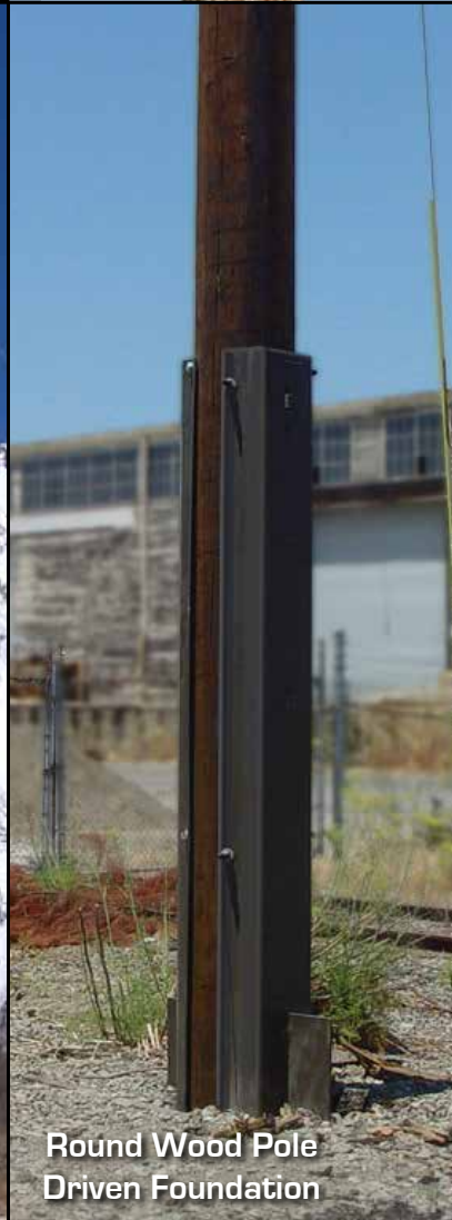
Woodpecker Damage Repair
