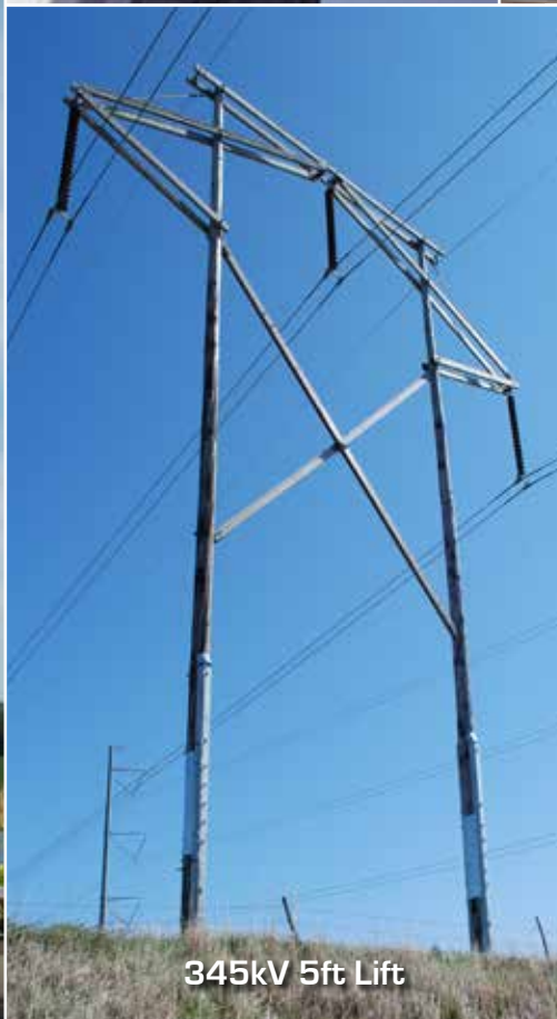
Cylinders Removed
