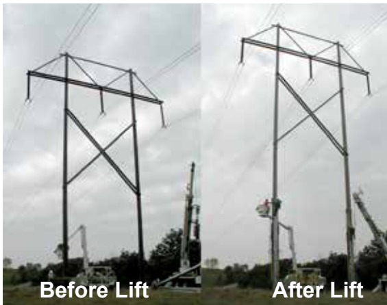
345kV H-frame structure raised 15 feet (Iowa)
