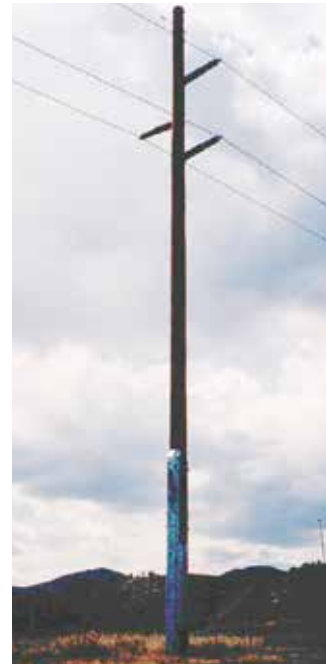
115kV Single Pole Structure Raised (& Reinforced) 10 feet - Alberta
