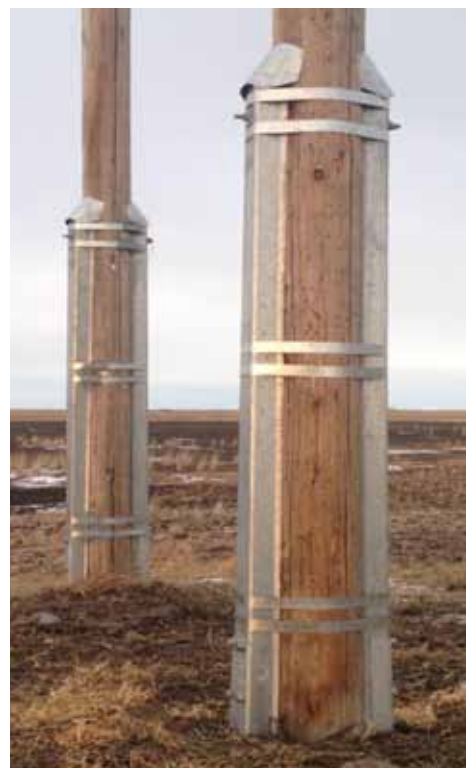
5. Units are banded and caps are installed.
