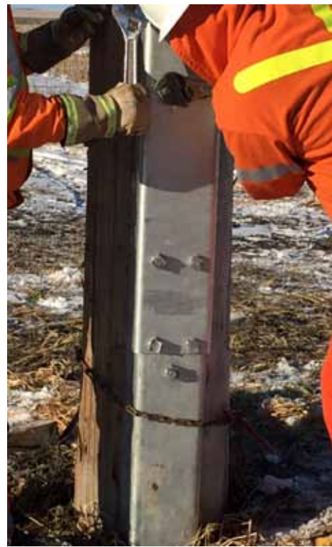
3. Top steel unit is attached and secured with splice channel.
