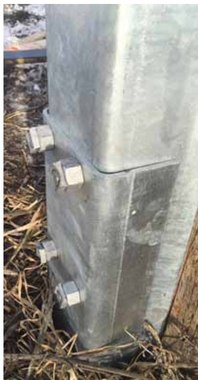
4. Assembled units are driven to desired depth.
