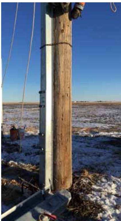
4. Assembled units are driven to desired depth.
