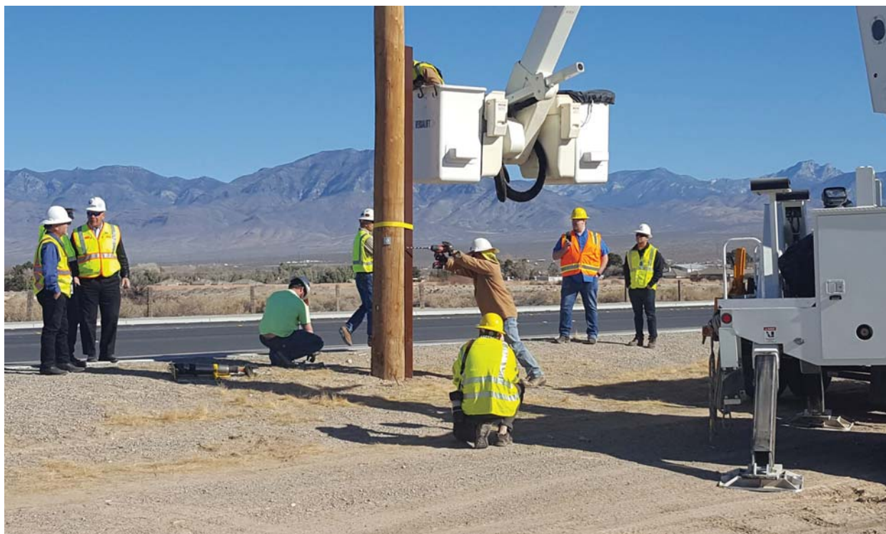
Valley Electric Association recently buttressed its poles to carry fiber.
